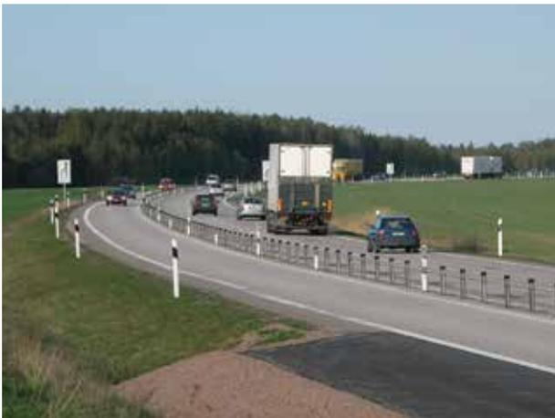
2+1 roads, which alternate two lanes on one side and one on the other every few kilometres, with a dividing barrier between, are part of Sweden's system-based approach to reducing the number of head-on crashes on highways.
