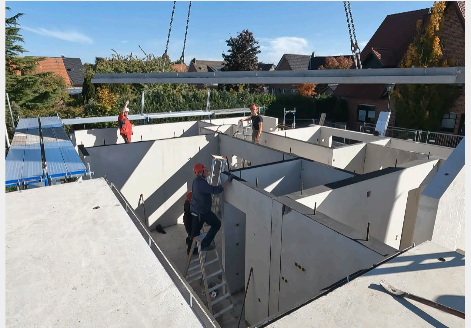
Image: Wall panels and concrete elements made from prefabricated concrete with recycled content in a residential building completed in 4 months [33].
