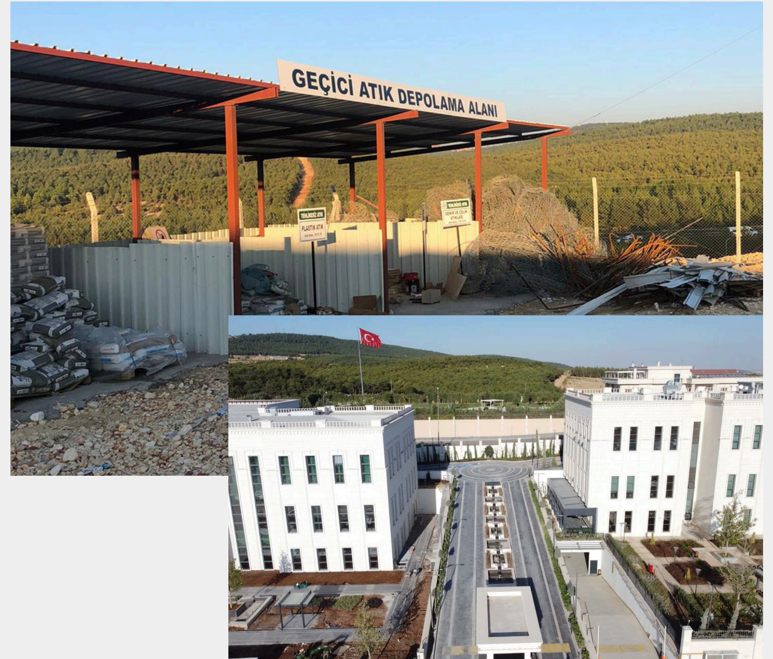
Image: The waste management area of the LEED Gold-certified SANKO Holding Gaziantep office building. During the construction process, 79.68% of the materials in nine different waste categories were recovered through recycling [35].
