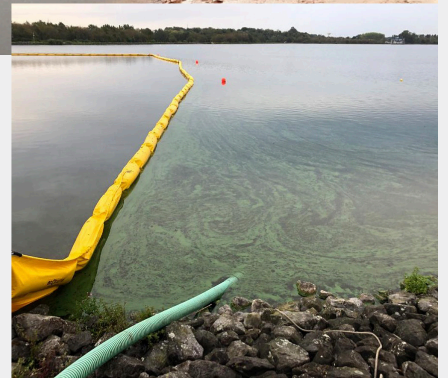
Image: The prevention of pollution from construction through water barriers [23].
