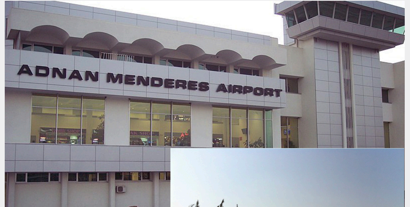
Image: The construction site buildings, parking lot shading elements, and all permanent construction site structures of the Izmir Adnan Menderes Airport Domestic Terminal were built entirely using salvaged building materials from the old airport structure [13].
