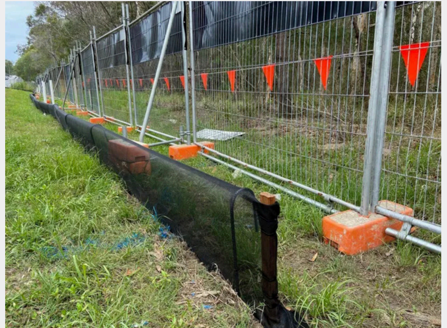
Image: Temporary fauna fence application. It prevents animal entry into the construction site and reduces live animal loss [27].
