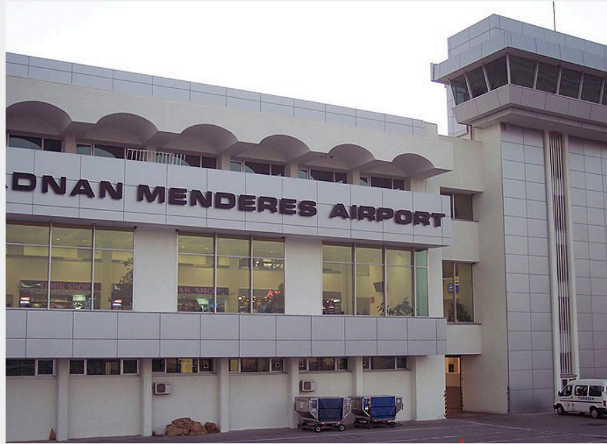
Image: The image depicts the demolished old İzmir Adnan Menderes Airport Domestic Terminal. With a planned approach, 95% of the demolished building was recycled [12].
