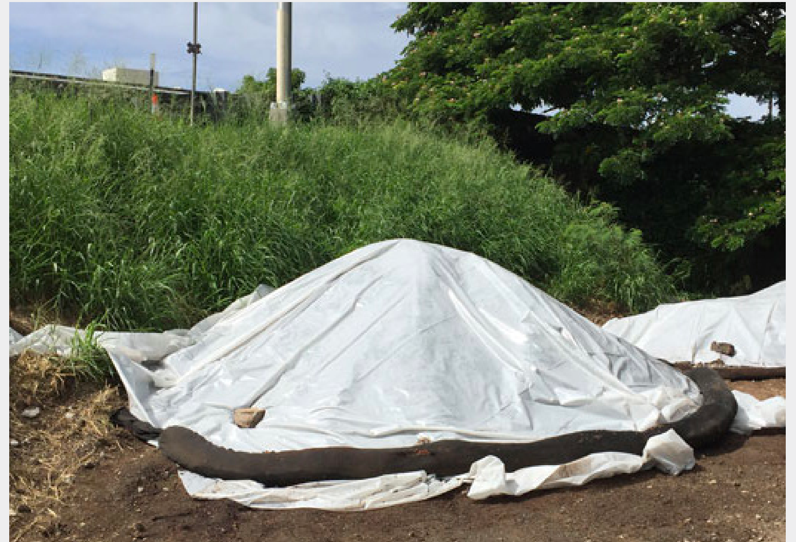
Image: The plant soil excavated from the construction site should be protected by covering it or temporary planting. Surface runoff should be prevented, and it should be reused in landscaping after construction is completed. [25]
