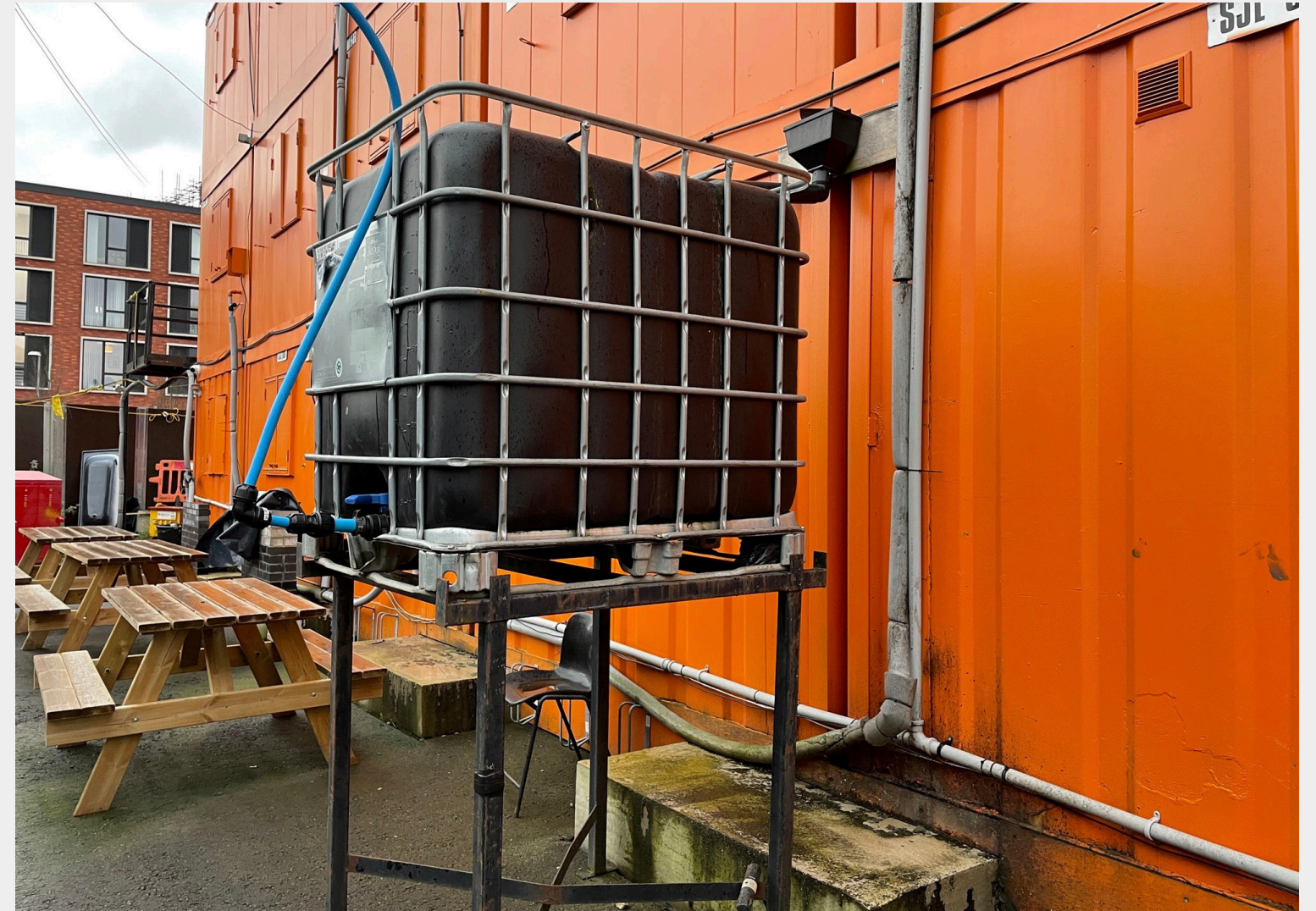
Image: Rainwater collected from the roofs of temporary structures on construction sites is used to wash vehicle tires [24].
