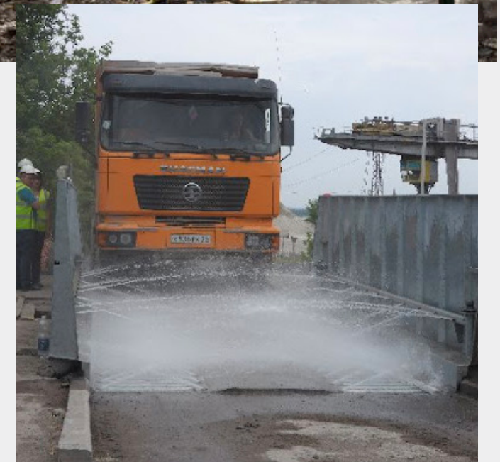
Visual: Cleaning of vehicle tires at the construction site exit [45].
