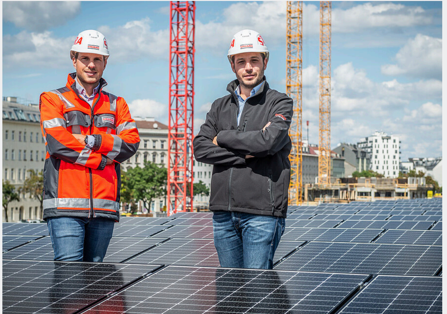
Image: In Vienna, Northern Railway Station site manager Daniel and technician Niko power their equipment and vehicles with green electricity generated from the rooftop of their site office. This approach not only saves energy but also reduces construction-related emissions [5].
