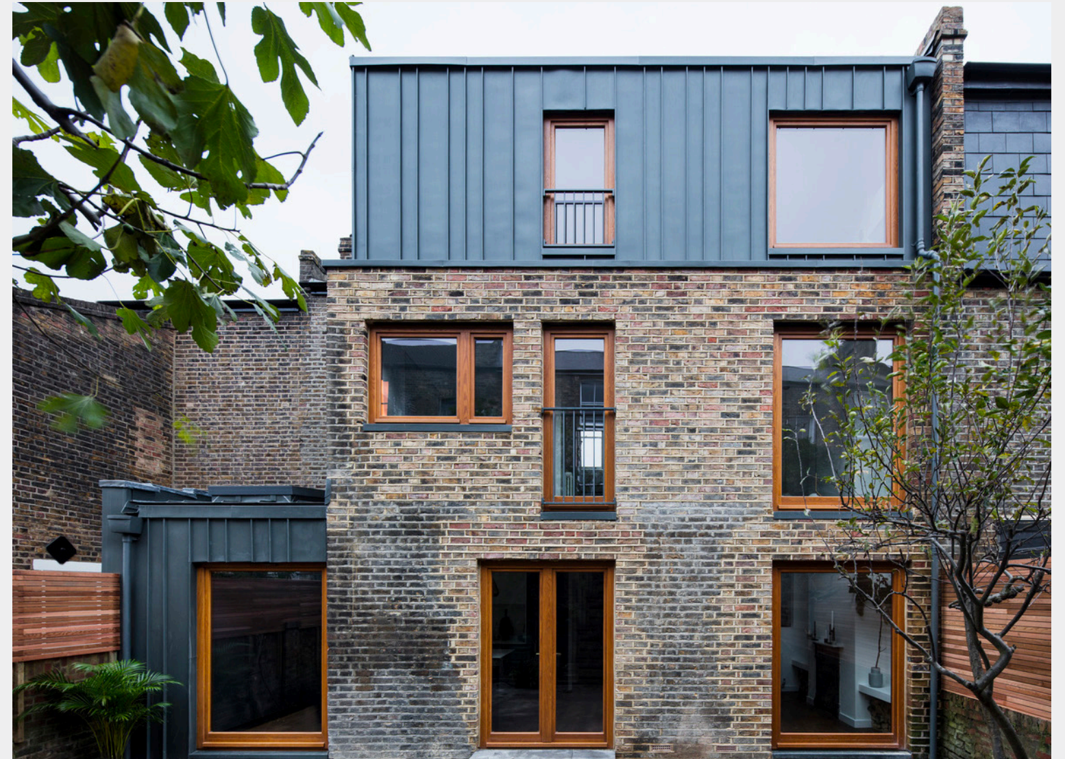
Image: A residential project built entirely from salvaged bricks and building materials. Elfort Road House / Amos Goldreich Architecture, London [34].
