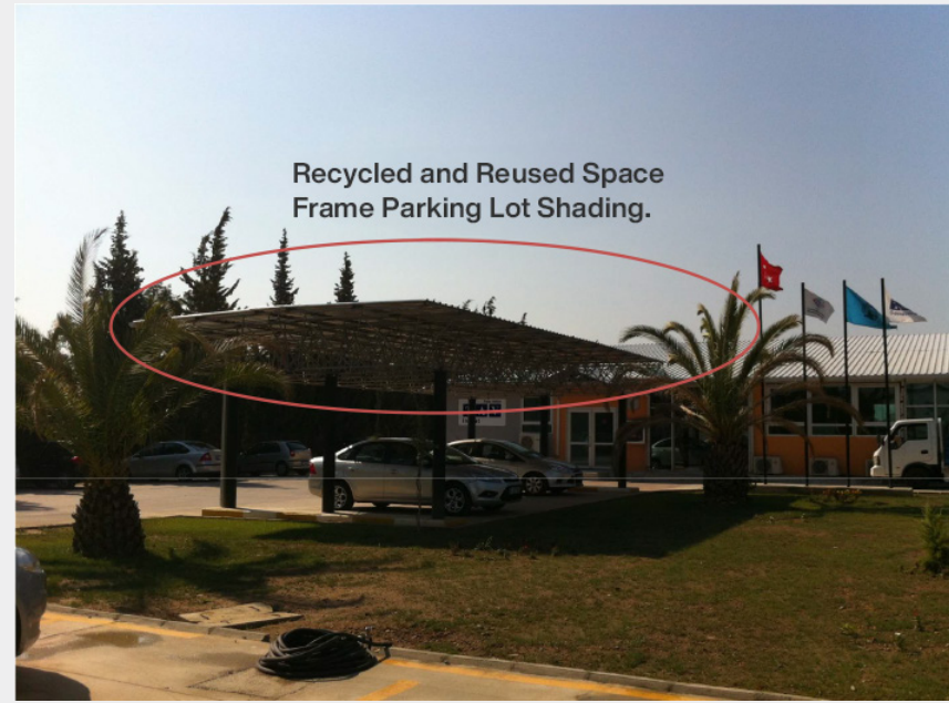
Image: Including the parking lot shading elements, 100% of the permanent construction site buildings were built using salvaged materials from the old airport structure [13].
