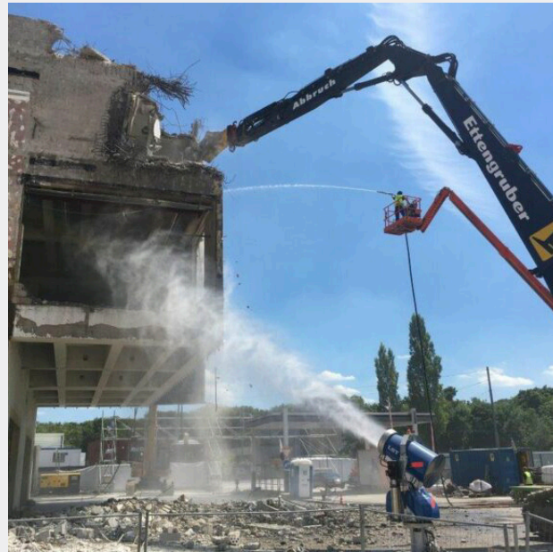
Dust control measures were implemented during demolition.
