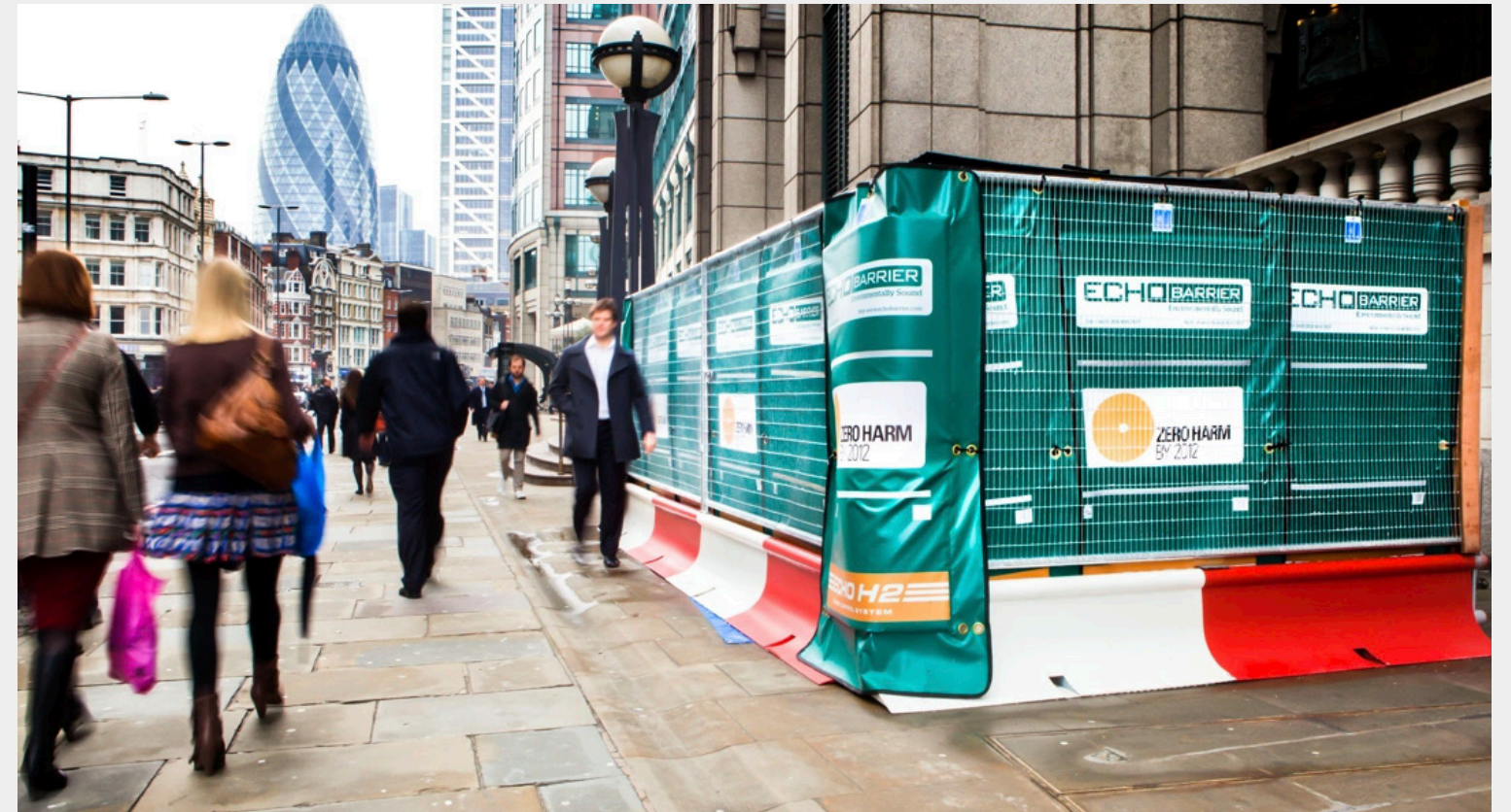
Image: Construction noise barrier in use, London [42].
