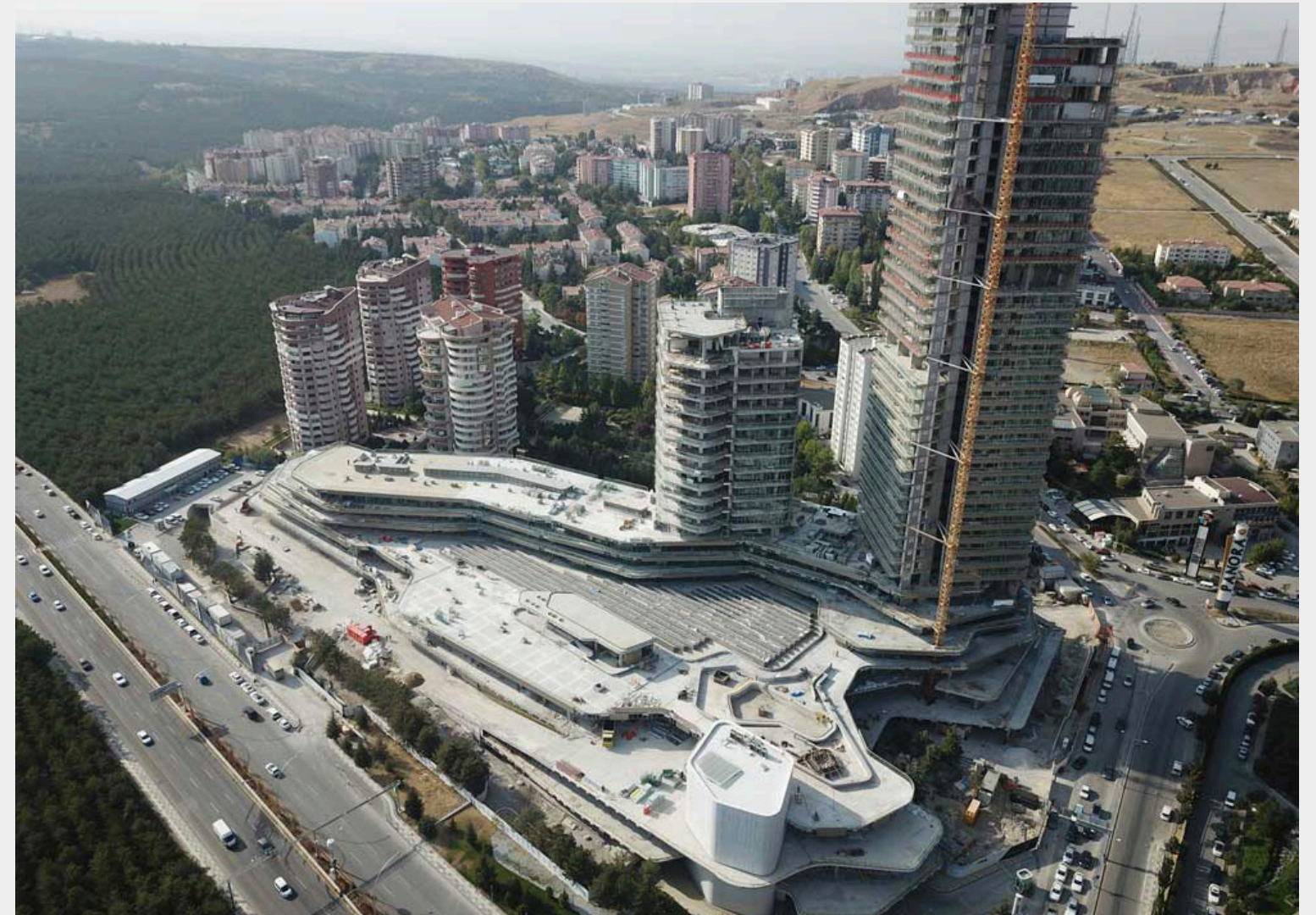
Image: The LEED Gold-certified Kuzu Effect Mixed-Use green building in Ankara has recycled 92% of its construction waste through its recycling practices [6].
