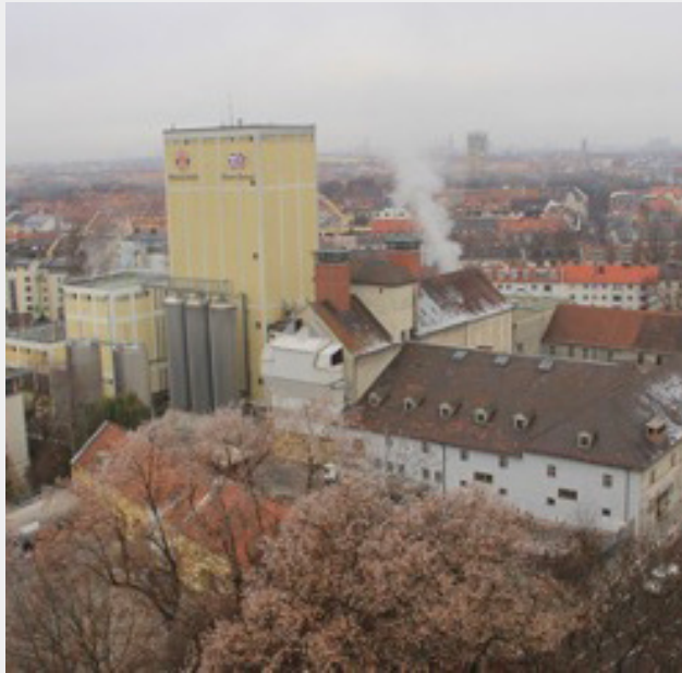
The former Paulaner Brewery in Munich Nockherberg was demolished using sustainable deconstruction techniques [56].
