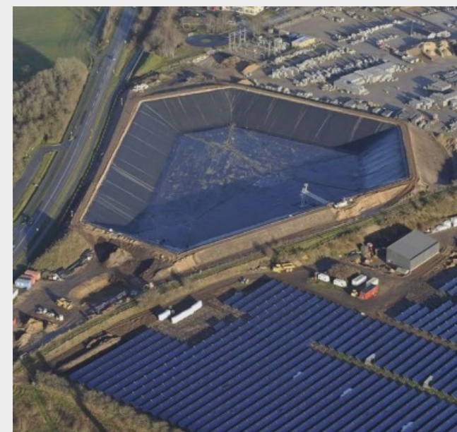
Seasonal thermal energy storage pit © Solmax
