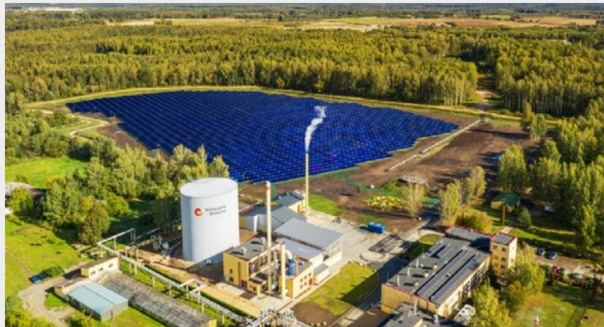
Salapis District Heating Plant
