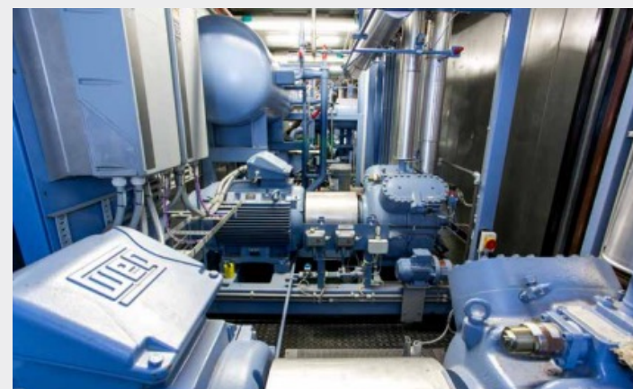
Two-Stage Ammonia Heat Pump
