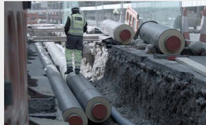
Bunhill Project Pipeline Installation
