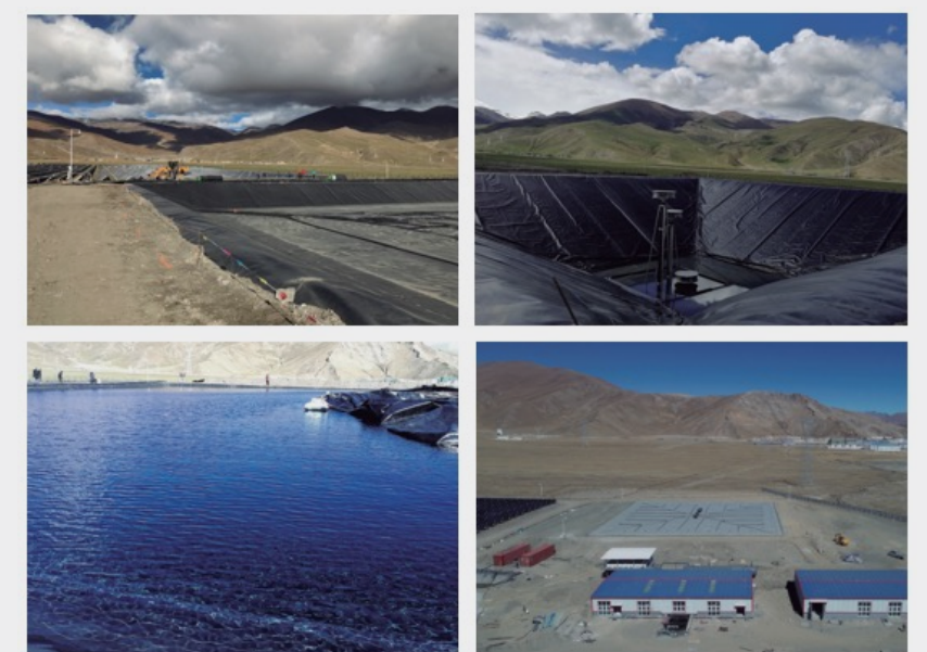
Seasonal storage fit construction © Arcon-Sunmark
