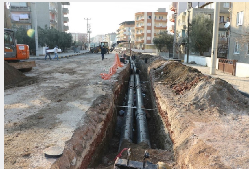
Soma District Heating System Pipeline Installation
