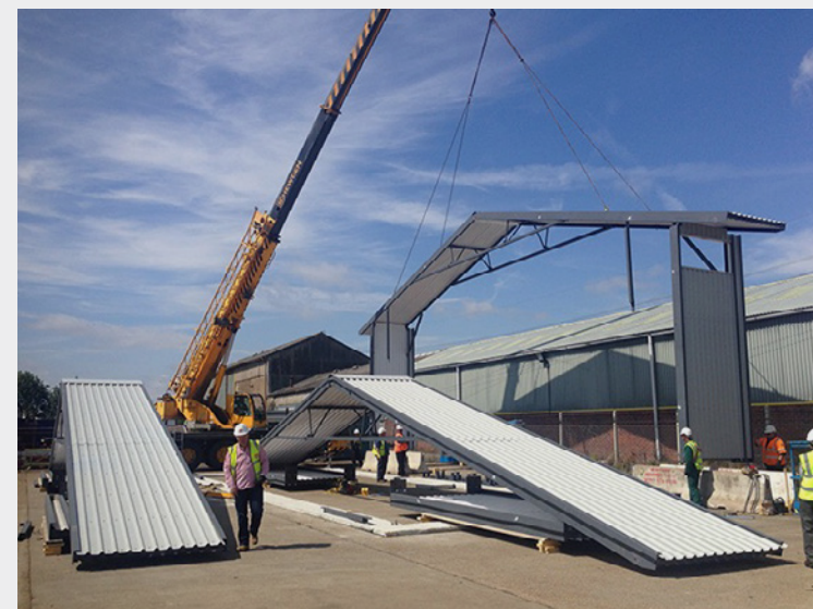
Assembly of the "Factory in a Box" prototype.
