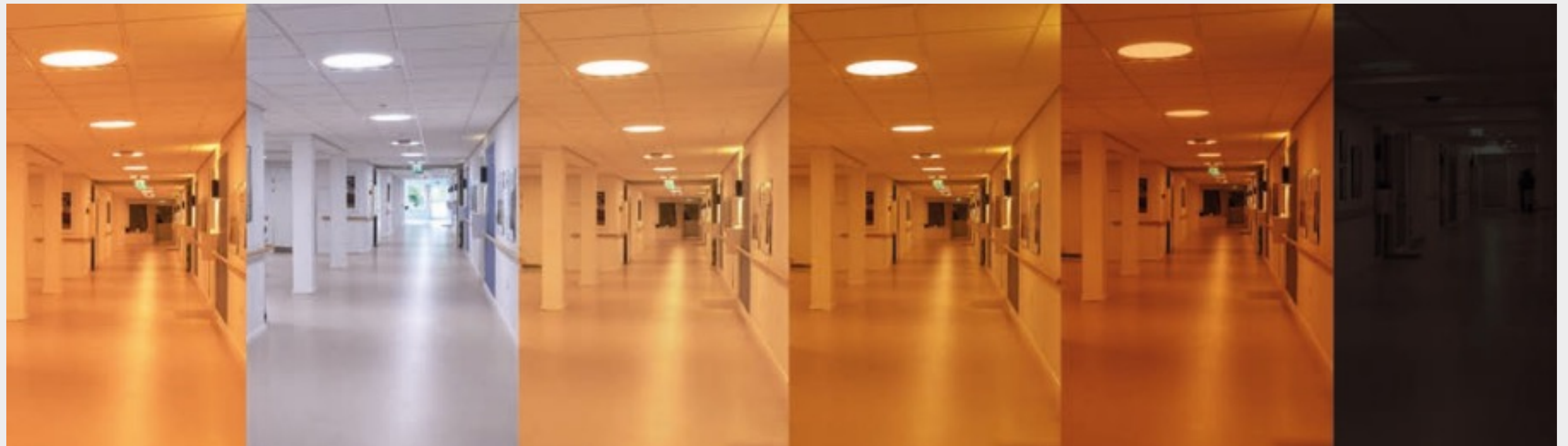
The lighting transitions smoothly throughout the day, from a gentle sunrise to bright daylight. In the afternoon, the light becomes warmer and gradually dims. During the night, patient rooms are kept dark, while common areas and corridors are equipped with night lighting that does not contain blue light @Chromaviso
