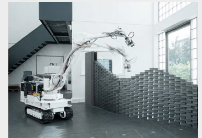
Brick-laying Robot © Gramazio Kohler Research, ETH Zurich
