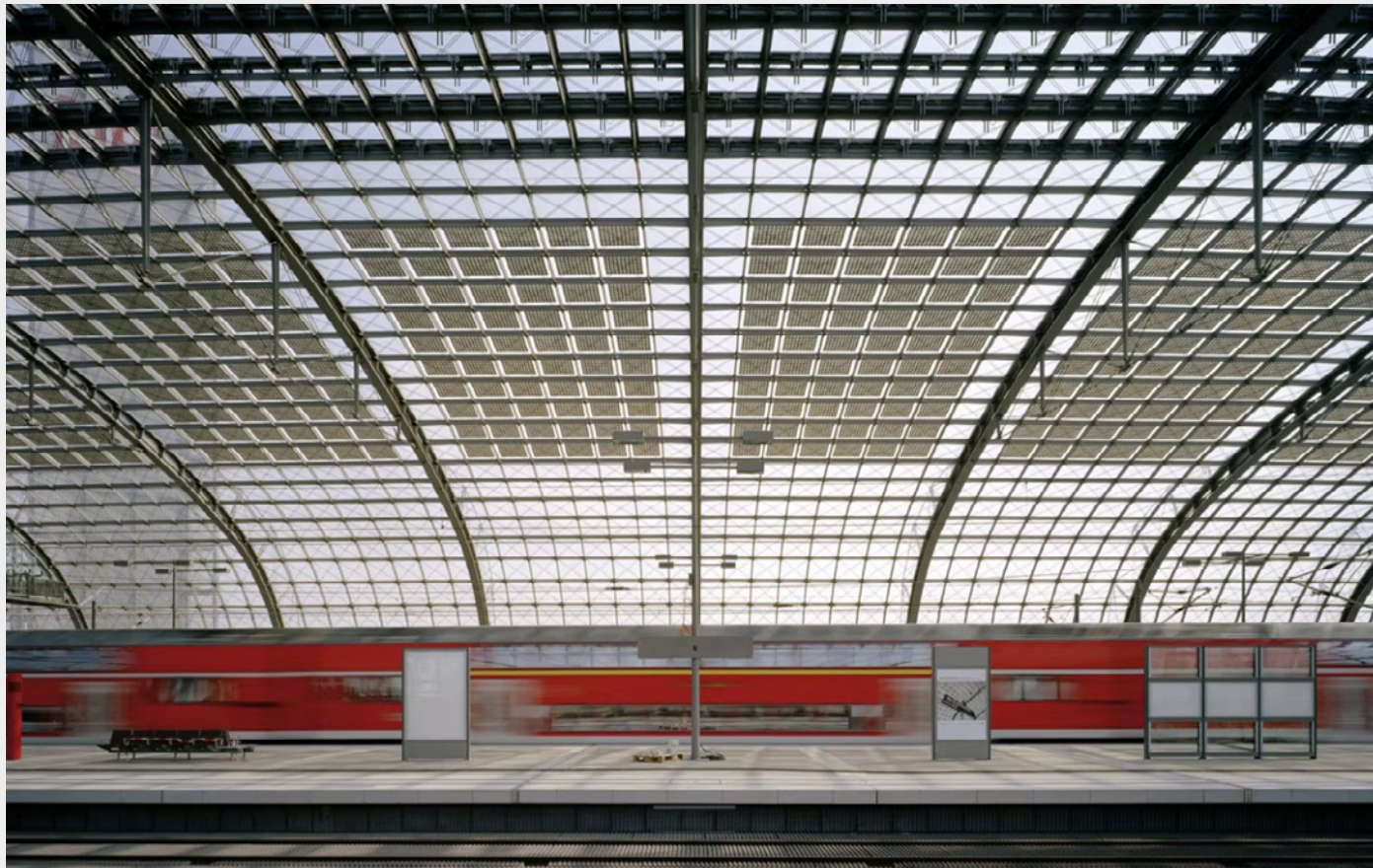
Photovoltaic Panels Integrated into the Station Roof
