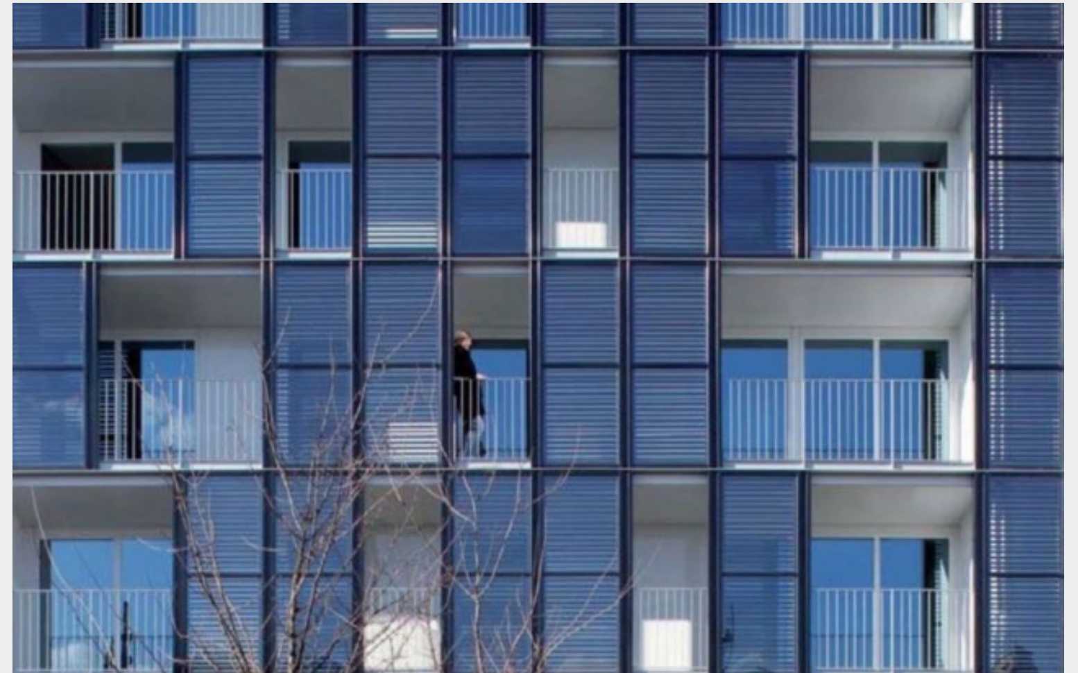
Vacuum Tube Solar Thermal Façade Application ©Philippon-Kalt Architectes
