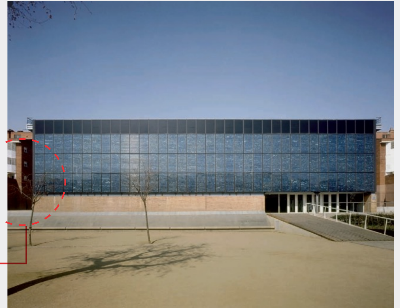
Pompeu Fabra Library's Naturally Ventilated Double-Skin Photovoltaic Façade
