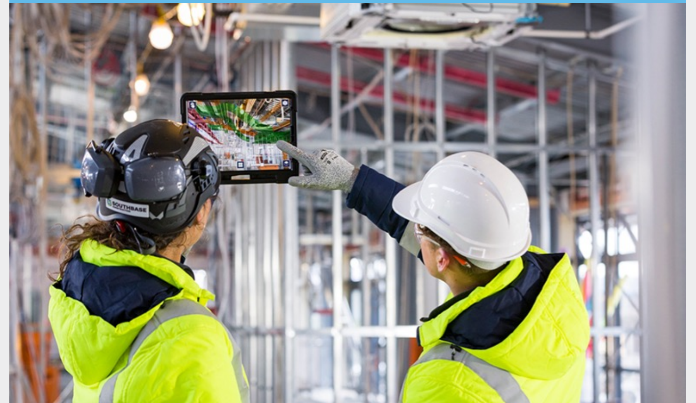
AR application on a mobile tablet at a construction ©Trimble
