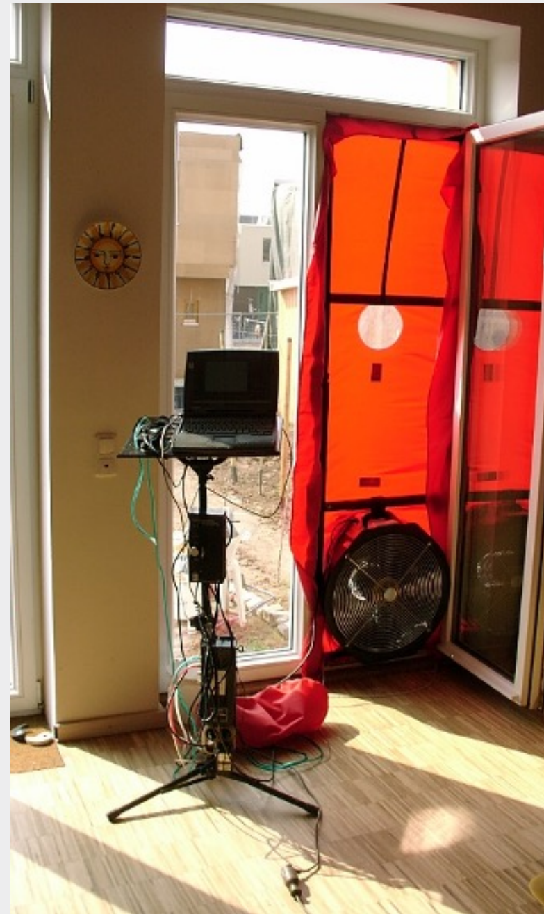
Airtightness Test Visuals in Passive House Buildings
